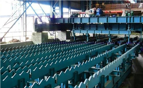
Turn over Cooling Bed
