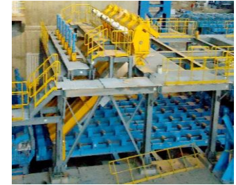
Steel Structure for Rigid Dummy Bar Storage Unit
