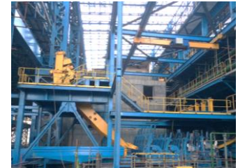
Steel Structure for WSU Unit
