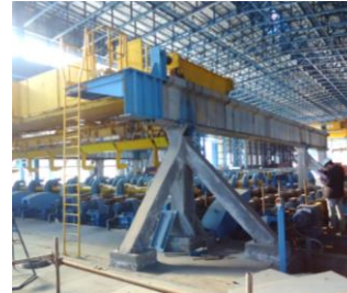
Support Structure for Cross Transfer Area
